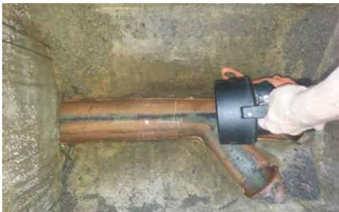
3. Rod the sewer or drain from the manhole or inspection chamber.
